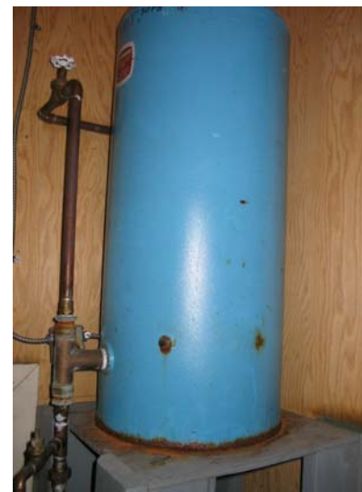
Photo 0022: 6542 Pressure Tank
