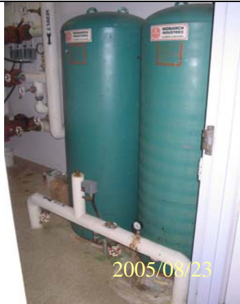
Photo 202: Water system. (pressure tanks & pump controls)
