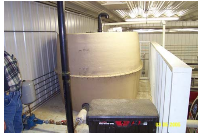
Photo 0066: 1953 Firehall 1250gal Water Storage Tank
