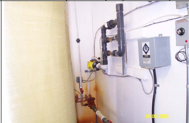
Photo 0070: 1953 Pumphouse Iron Duplex Injection Chlorine System
