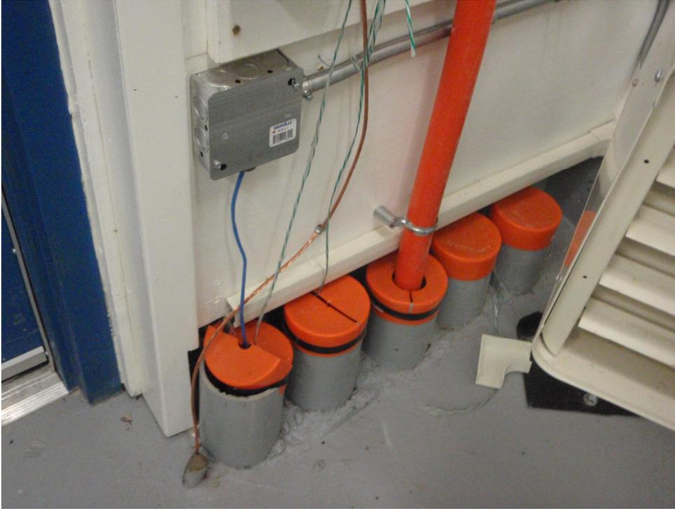
**Figure 10** Photo showing poorly sealed electrical and cable conduits in Wellhouse . If a flood occurred in the wellhouse water could enter the aquifer after entering conduits.
