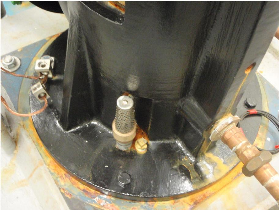
**Figure** Photo of the well head of Well . This shows a secured well head sealed from potential flooding with a check valve on the air vent and a bolted nut for manual water level access.
