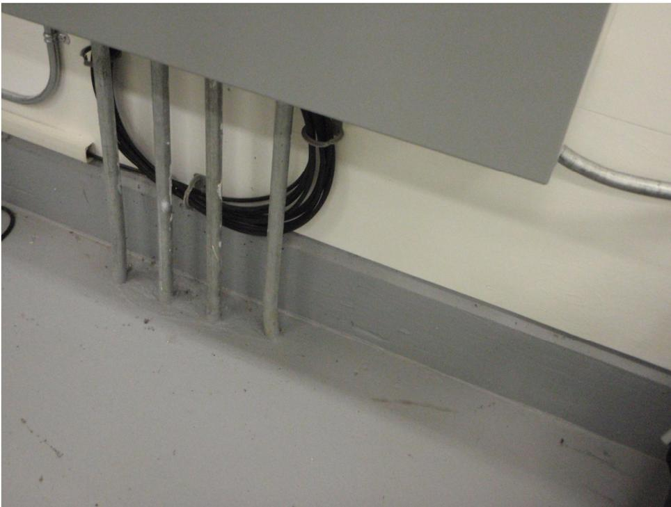
**Figure 11** Photo showing well-sealed electrical conduits in Wellhouse .
