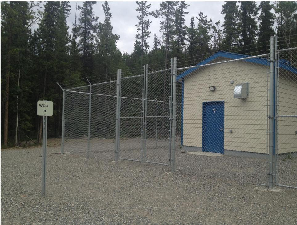
**Figure 6 Photo of Well 9 Wellhouse. Notice the slight downhill slope away from the wellhouse which provides good drainage away from the building in the event of a flood in the wellhouse. Well 9 Wellhouse is similar as it was completed at the same time.**
