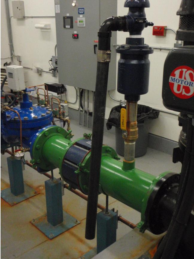
**Figure** Photo showing the air vent on Well . Note no backflow preventer. In the event of a flood the water would be sucked back into the well. We understand the City of Whitehorse has since cut off the length of the air vent to near the top and installed a flood alarm about 0.3m above floor level.
