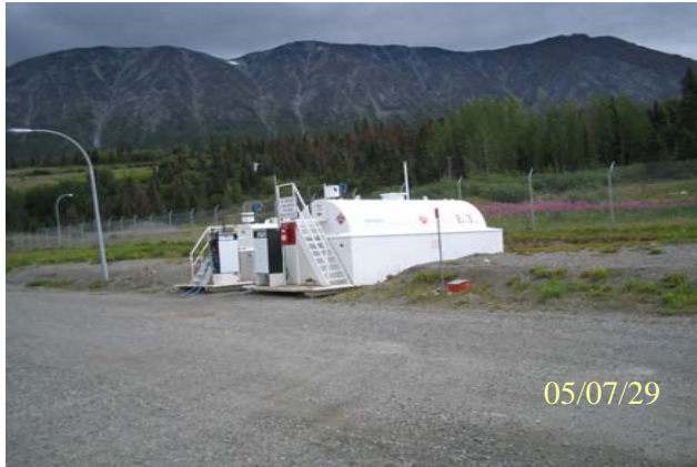
Photo 0137: 3440 Above ground fuel storage tank
