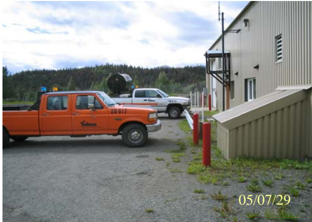
Photo 0139: 3440 Blanchard Grader Station maintenance garage
