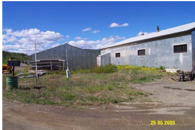
Photo 0205: 6512 Septic Field and Rock Pit (left), Carmacks Grader Station (back right)
