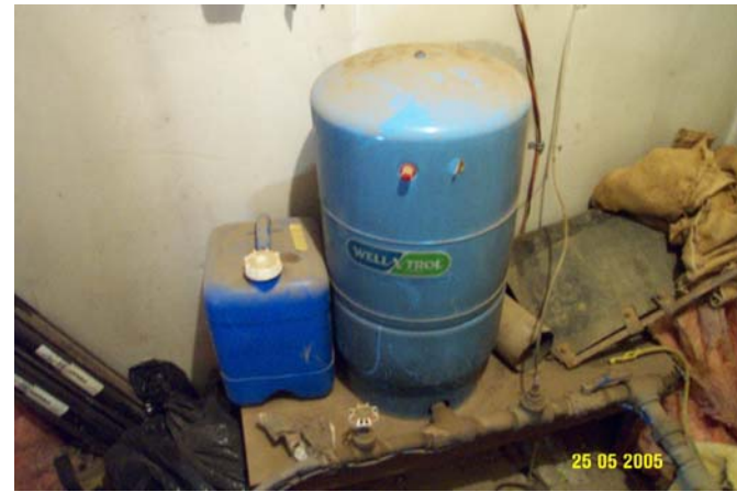
Photo 0198: 6512 Pressure Tank
