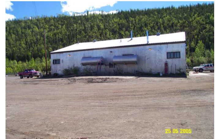
Photo 0202: 6512 Above Ground Fuel Storage Tanks (2) and Carmacks Grader Station (behind)
