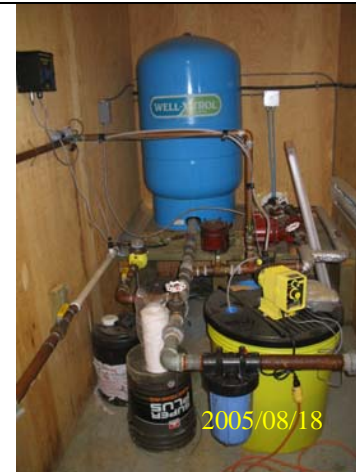
Photo 174: 5690 water system that serves 5681 & 5682. (pressure tank, filter, pump controls, LMI proportion feed chlorination system).
