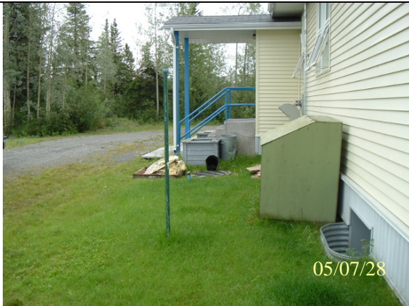
Photo 0567: 3100 Wellhead in pit (back centre), underground fuel storage tank (front centre), school (right)
