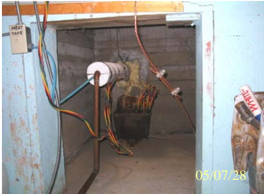
Photo 0101: 3100 Point of entry from well (top), abandoned well under box (bottom)
