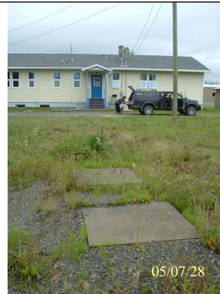
Photo 0569: 3100 Septic tank (front), school (rear)
