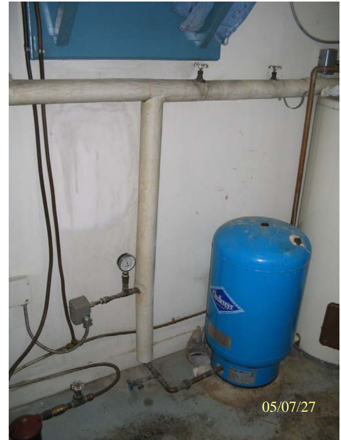
Photo 0074: 3123 Pressure tank and pump controls
