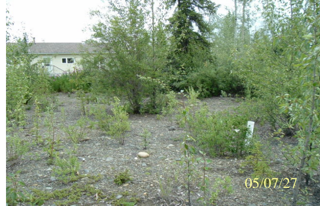
Photo 0547: M0134 Septic field looking east towards residence
