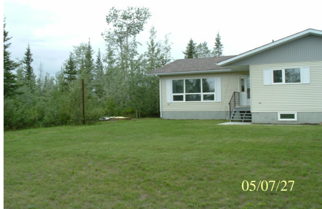
Photo 0549: M0134 Beaver Creek RCMP Residence (right), wellhead enclosure (left)
