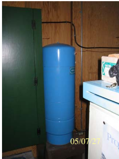
Photo 0077: 3964 Pressure tank
