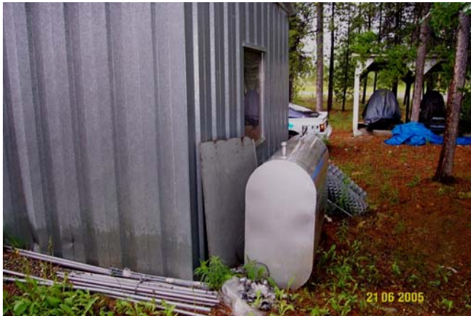
Photo 0285: M0084 (RCMP gym, left) Above ground fuel storage tank (centre)
