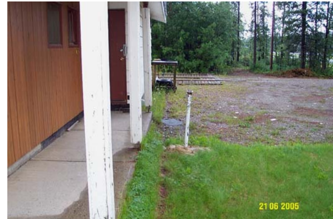
Photo 0283: M0092 Potential underground fuel storage tank (centre), RCMP detachment building (left)
