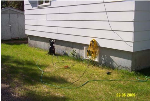
Photo 0306: M0086 Watson Lake RCMP Residence – location of well off of basement
