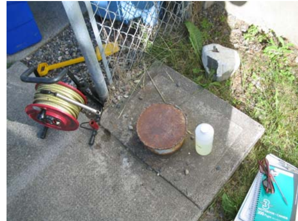
Photo 0037: M0088 Well casing extended above grade – not connected to casing below
