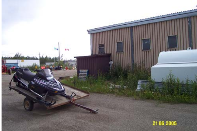
Photo 0273: 4836 Grader Storage Building and wellhead enclosure addition (back), above ground fuel storage tank (right)
