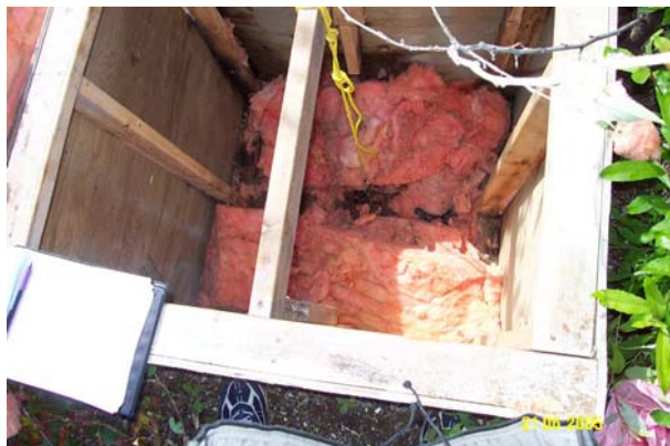
Photo 0240: 4842 Wellhead in pit
