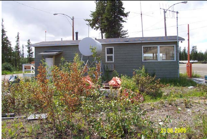
Photo 0238: 4842 Cassiar Weigh Scales (back), wellhead enclosure (centre), above ground fuel storage tank (left centre), water storage tank for kitchen cold water tap (left)
