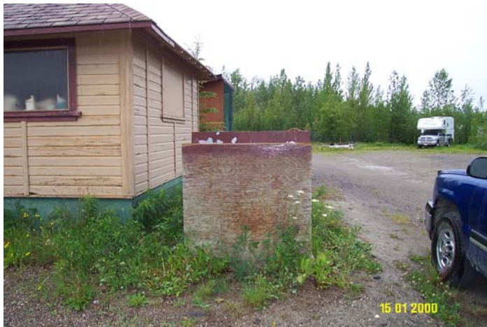
Photo 0261: 4840 Wellhead enclosure (centre), and storage building (back left)
