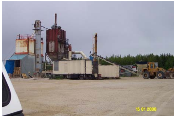
Photo 0266: Barite ore storage lot south and likely up gradient from 4840 well
