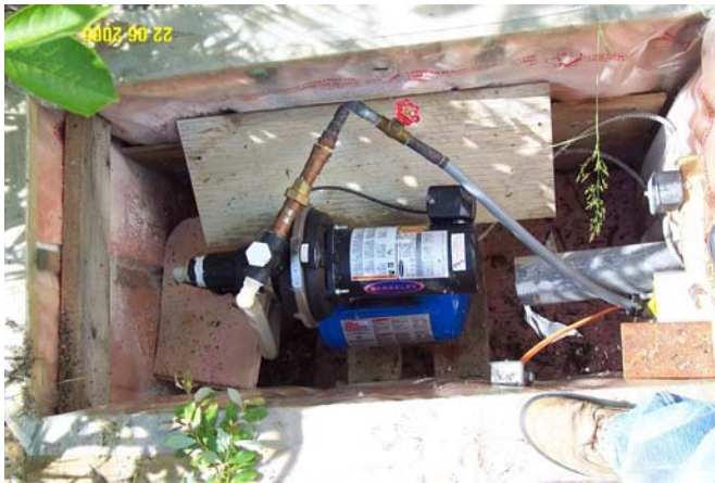
Photo 0308: 4976 Wellhead in pit (left), and jet pump (centre)
