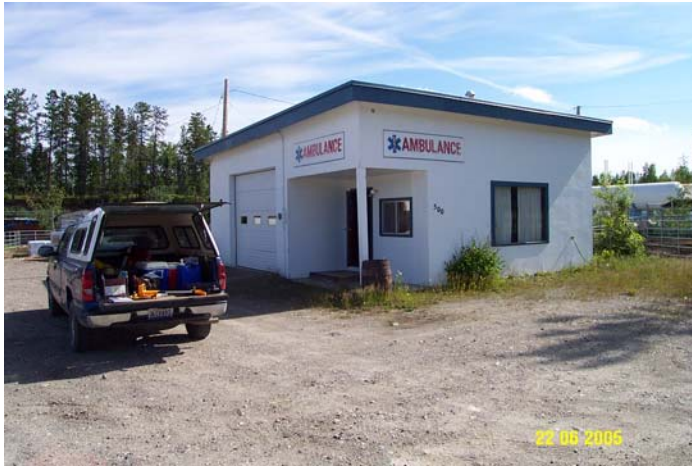
Photo 0312: 4976 Watson Lake Ambulance Building
