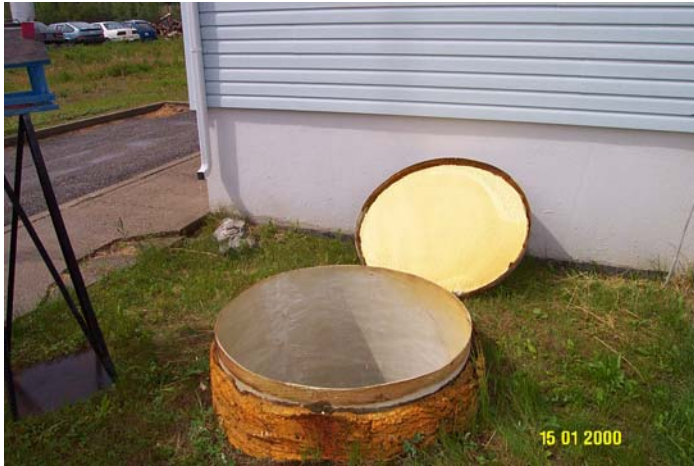
Photo 0270: 4981 Wellhead enclosure (front), and EMR office (behind)
