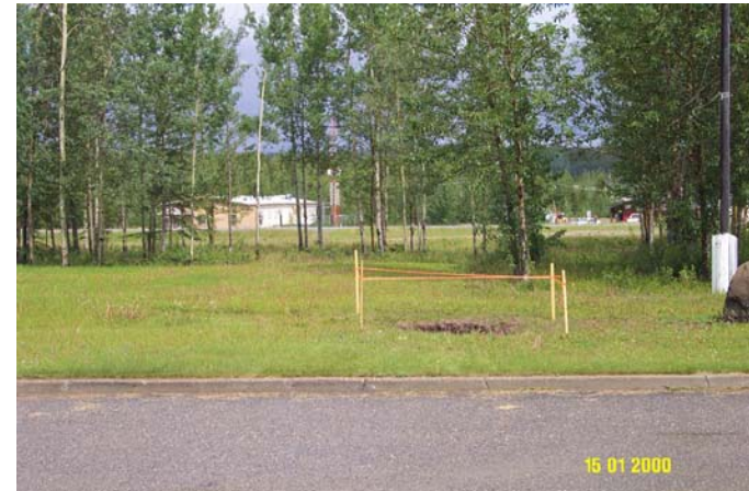
Photo 0267: 4981 Sinkhole – could be abandoned septic tank
