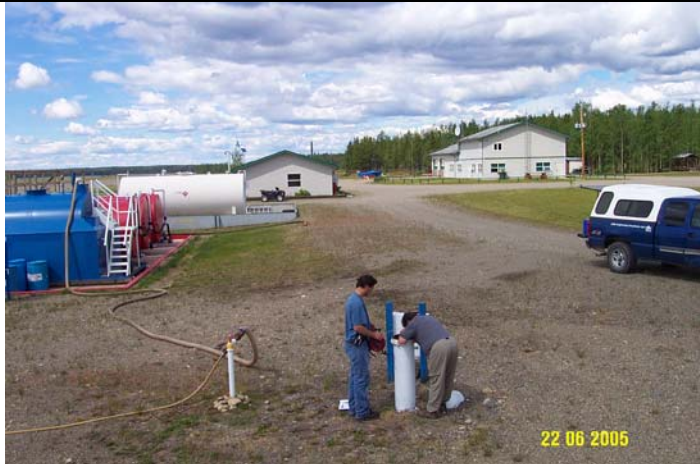
Photo 0319: 4993/4994 Pitless unit (front centre), EMR Fire Control Centre (4993, back right), EMR Tanker Base (4994, back centre), above ground fuel storage and fire retardant tanks (left)
