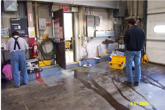
Photo 0232: 4793 Wellhead in maintenance garage
