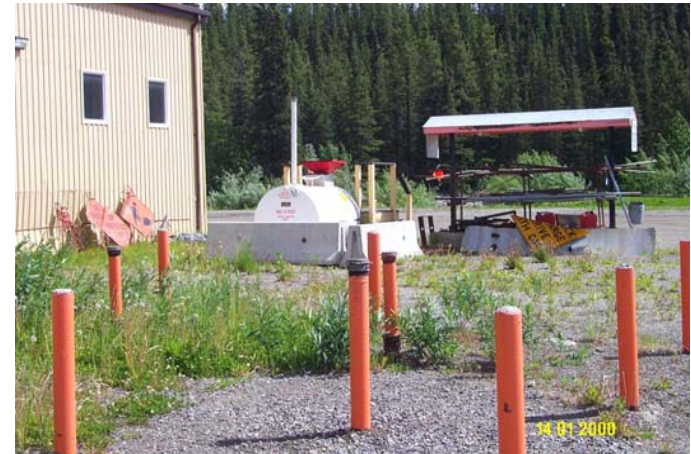
Photo 0236: 4793 Underground fuel storage tank nest (front), used oil tank (back), maintenance garage (back left)
