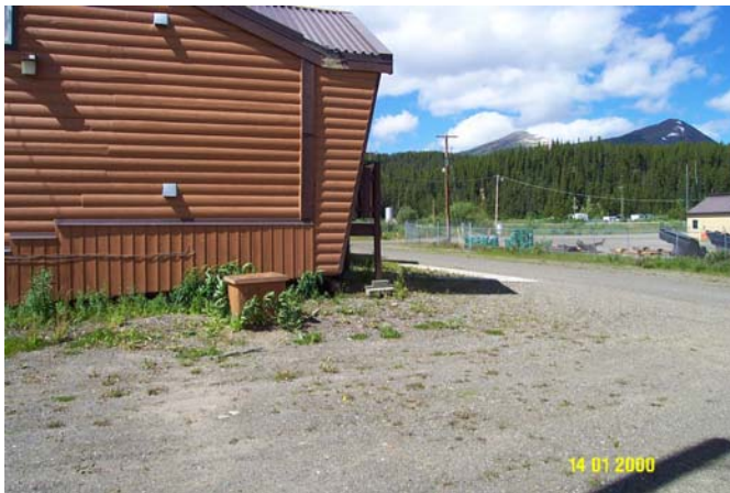
Photo 0240: 4799 Swift River Living Complex (back) and wellhead enclosure (in front)
