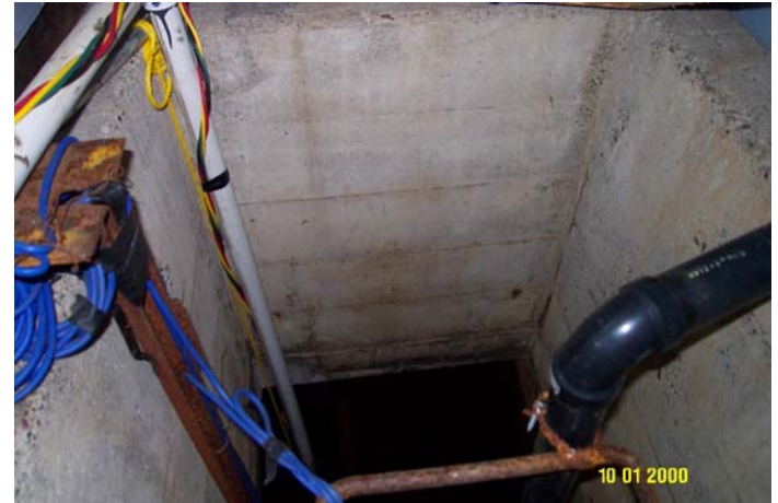
Photo 0220: 4782 Cistern inside Water Reservoir building
