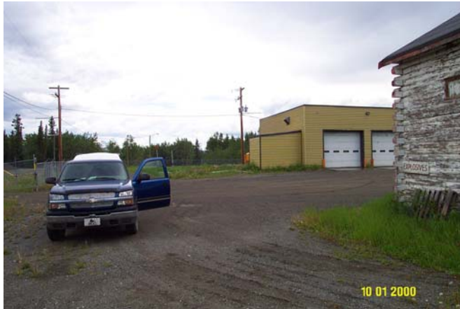
Photo 0222: 4782 Teslin Grader Station (back) and Water Reservoir building (right)
