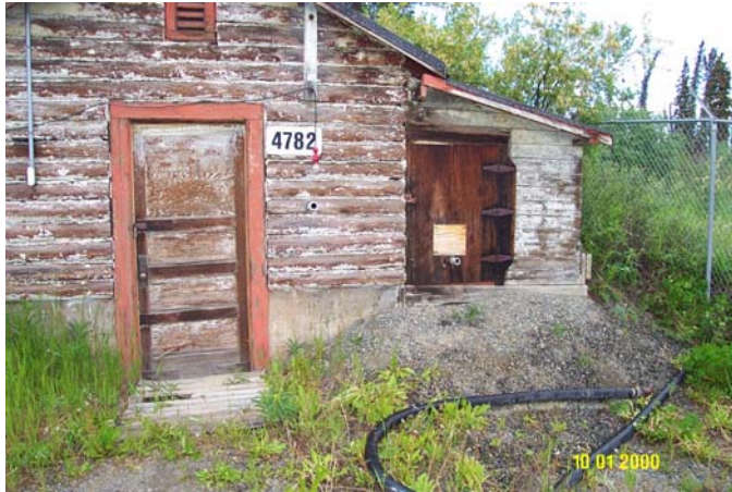
Photo 0218: 4782 Water Reservoir building
