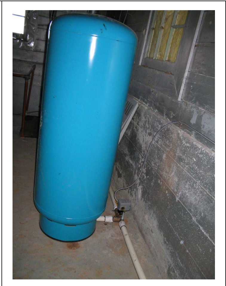
Photo 0009: 4782 Pressure tank
