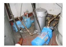
Photo 0495: 1134 Jet Pumps and Tank
