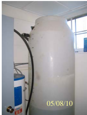
Photo 141: 1131 Water storage tank.
