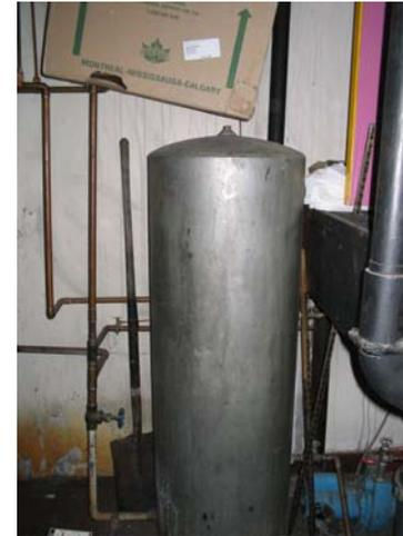
**Photo 0498:** 1134 Potable Water Pressure Tank
