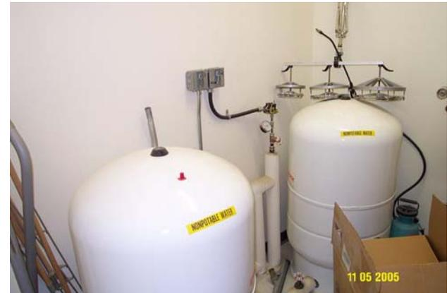
**Photo 122:** 1134 Pressure Tanks and Flow Switch
