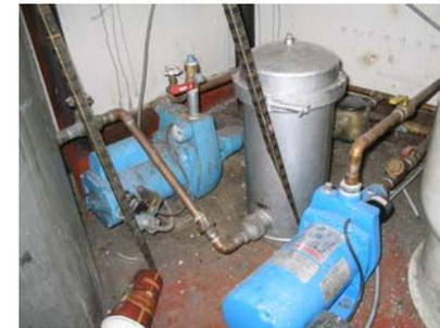
**Photo 0495:** 1134 Jet Pumps and Tank
