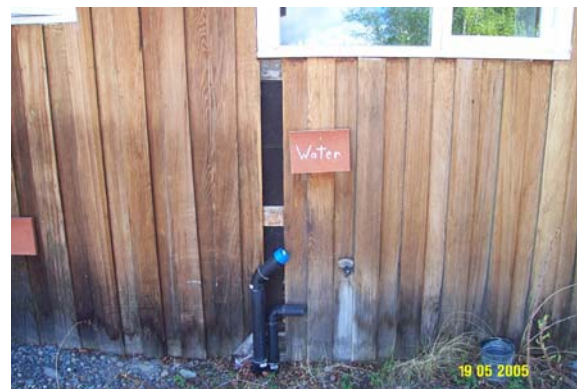
Photo 0184: YWP-B Trucked Water Intake
