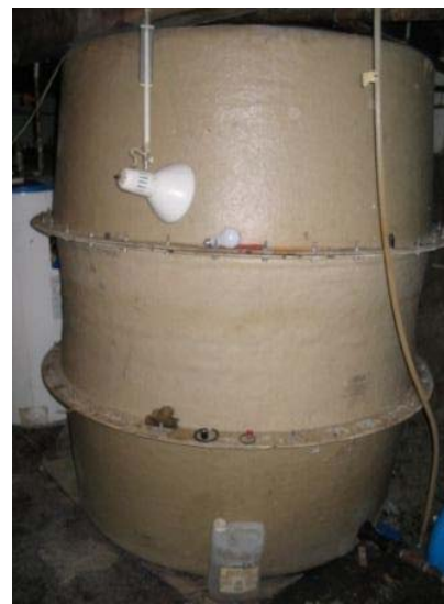
Photo 0006: YWP-B Trucked Water Storage Tank
