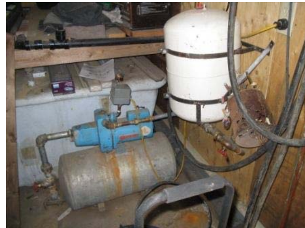
Photo 0184: YWP-D Jet Pump and Pressure Tank
