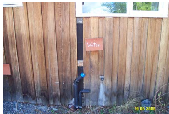
Photo 0184: YWP-B Trucked Water Intake
