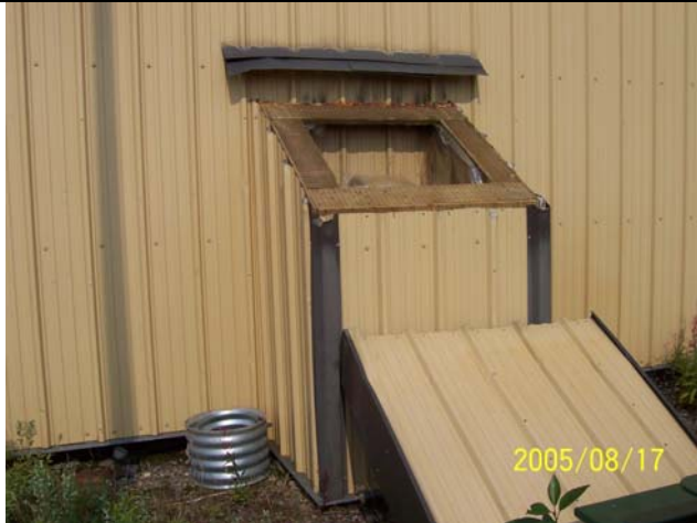
Photo 044: 5629 Wellhead enclosure.
