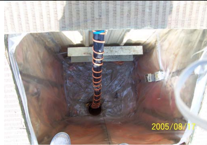
Photo 033: 5629 Well enclosure and wellhead in pit.
