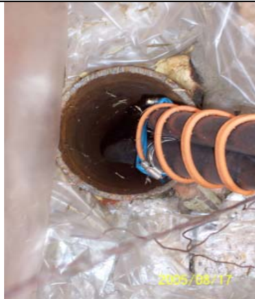
Photo 042: 5629 Wellhead – note that there was no well cap at the time of assessment.
