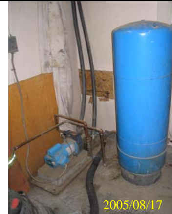
Photo 192: 5629 Grader station pressure tank and jet pump.
