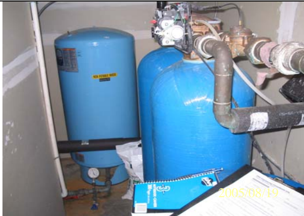
Photo 230: 2599 Pressure tank, pump controls and softener system.
