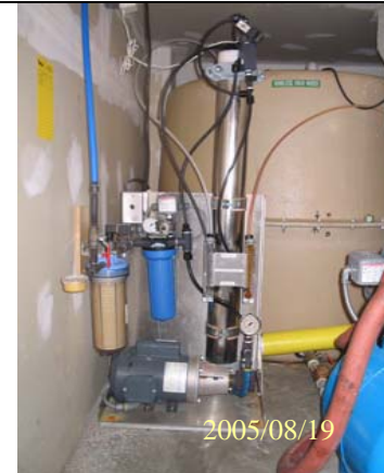
Photo 234: 2599 Reverse osmosis system (front) water storage tank (back)
