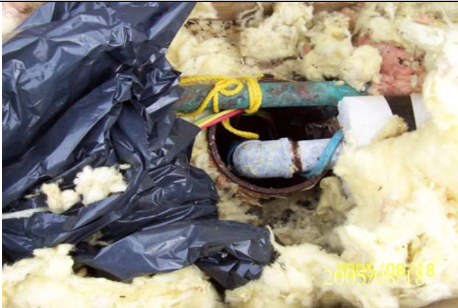
Photo 065: 2600 Wellhead – note that at the time of the assessment there was no well cap and evidence of mice around the wellhead.
