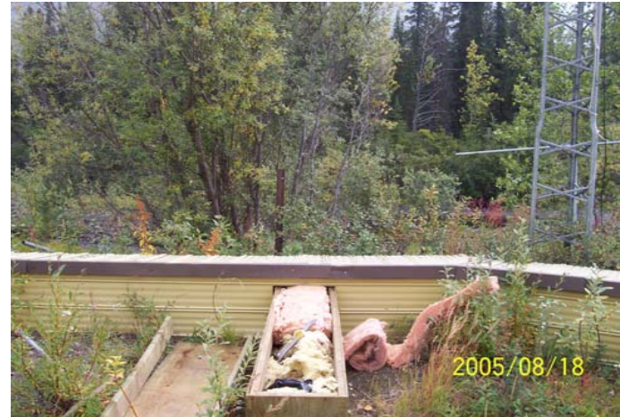
Photo 067: 2600 Wellhead with surrounding enclosure and utilidor.
