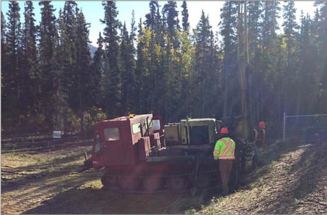
Photo 3: Setting up the drill rig at borehole location 15BH01.
