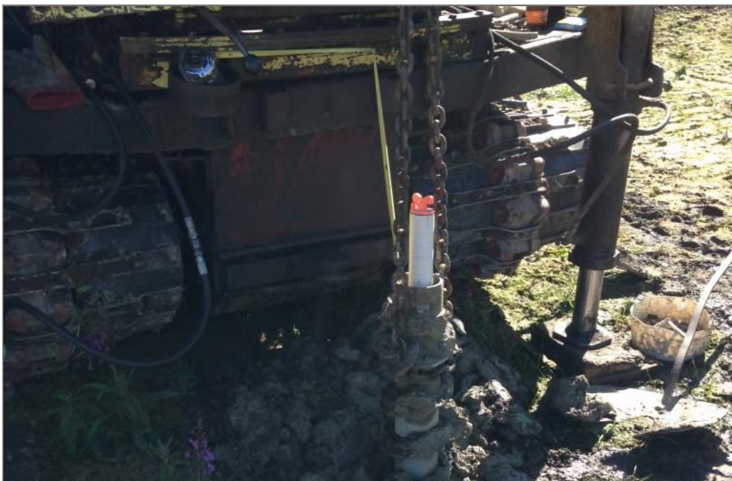
Photo 4: Installation of 15MW01.
