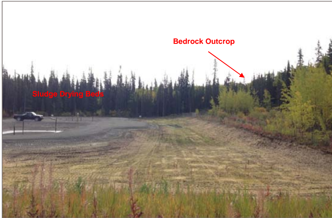
Photo 1: Hydroseeded area south of the sludge drying beds, looking southeast.
