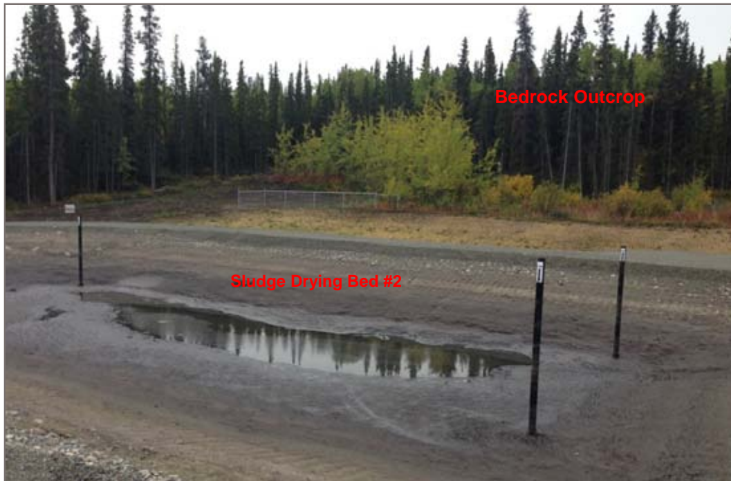
Photo 2: Sludge drying bed #2, looking southeast. Bedrock outcrop was noted behind the fence.
