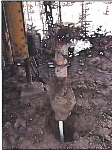
Photo 1. Well casing and protective casing removal at GW4
