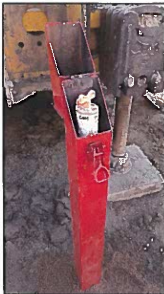
Photo 5. Completed monitoring well (GW4-2019)
