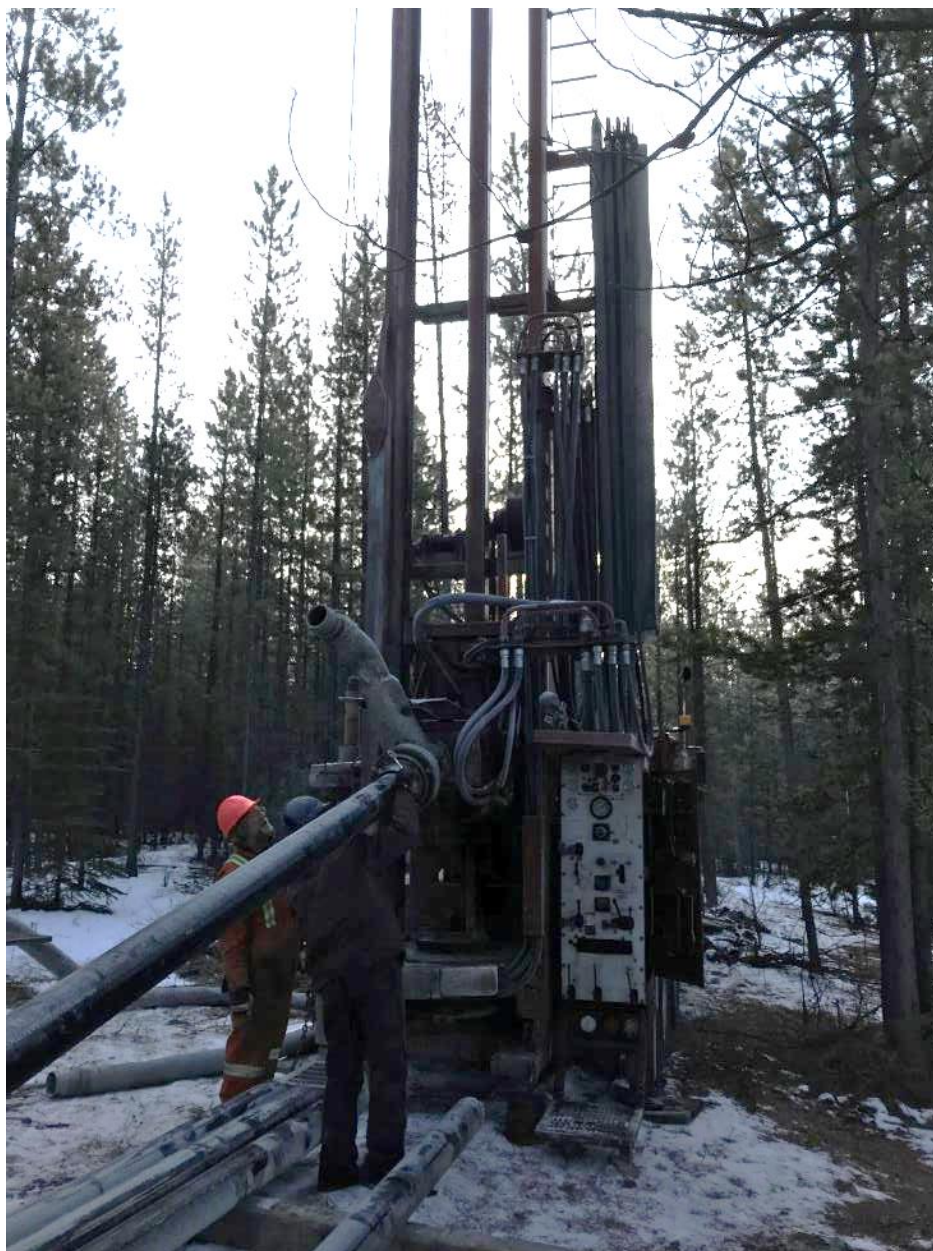
Photo 3: Air-rotary drill rig at MW1-19, Impact Well Drilling. (22 October 2019)
