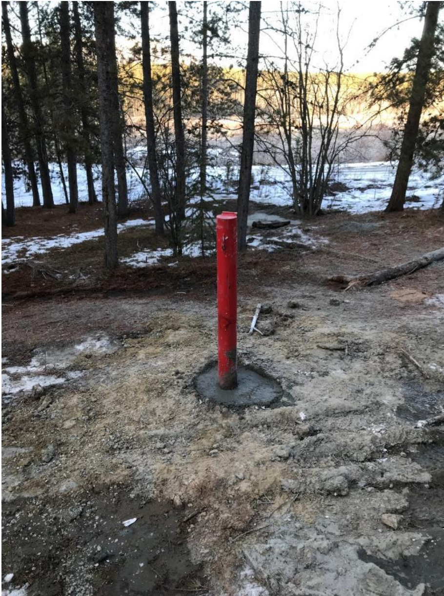
Photo 7: Completed Monitoring Well MW1-19. (25 October 2019)
